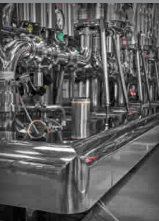
Enclosed perimeter channel with casing
