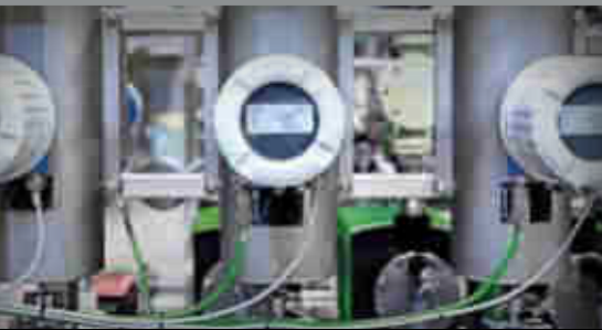
Large injection dosing units
