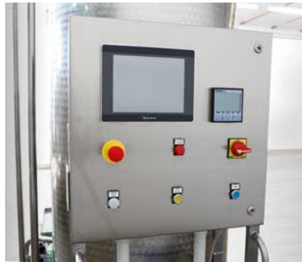
ELECTRICAL PANEL WITH pH METER
